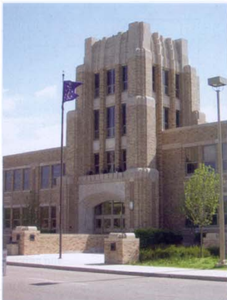
Main tower entry (After)
